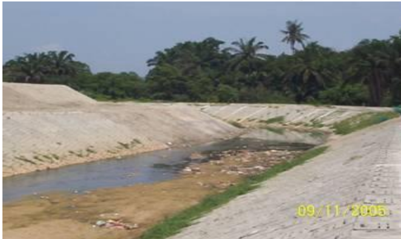
Sg. Rajah with flex-slab lining
