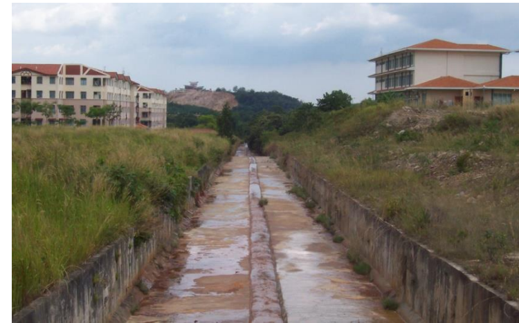
Sg. KFC Flood Mitigation – Existing Concrete lined River
