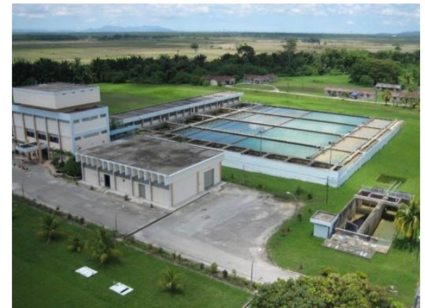
Teluk Kepayang Water Treatment Plant
