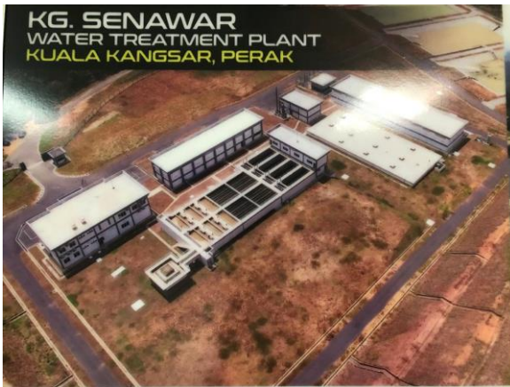
Kuala Kangsar Water Treatment Plant
