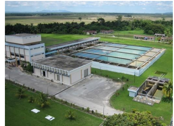
Teluk Kepayang Water Treatment Plant
