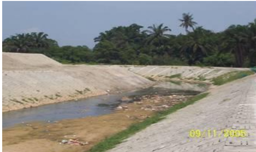
Sg. Rajah with flex-slab lining
