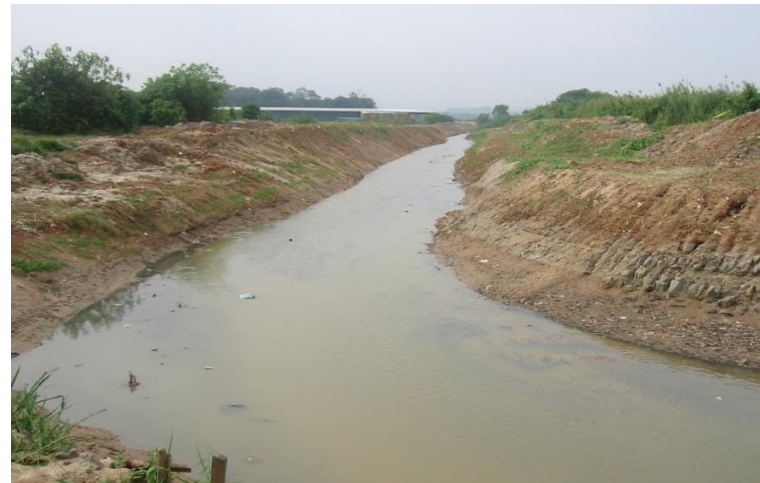
Sg. Rajah Improvement Works
