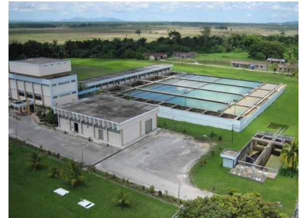
Teluk Kepayang Water Treatment Plant
