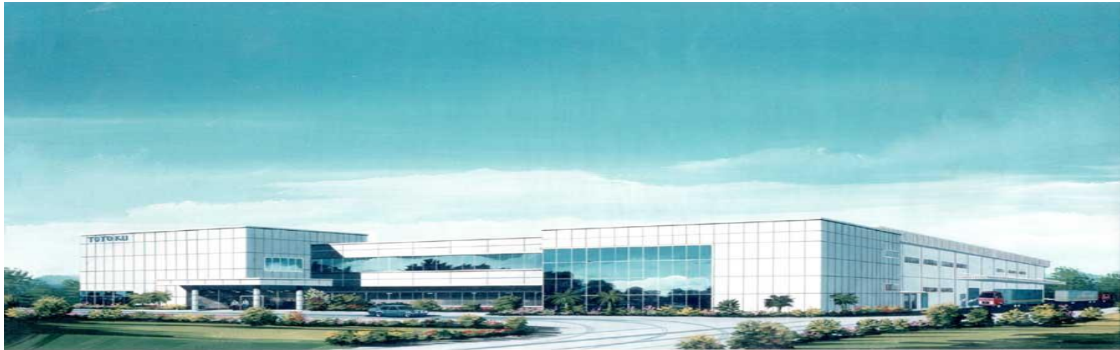
Double storey factory and administration block at Bukit Raja Prime Industrial Park, Kapar, Klang For M/s Totoku (M) Sdn. Bhd.
