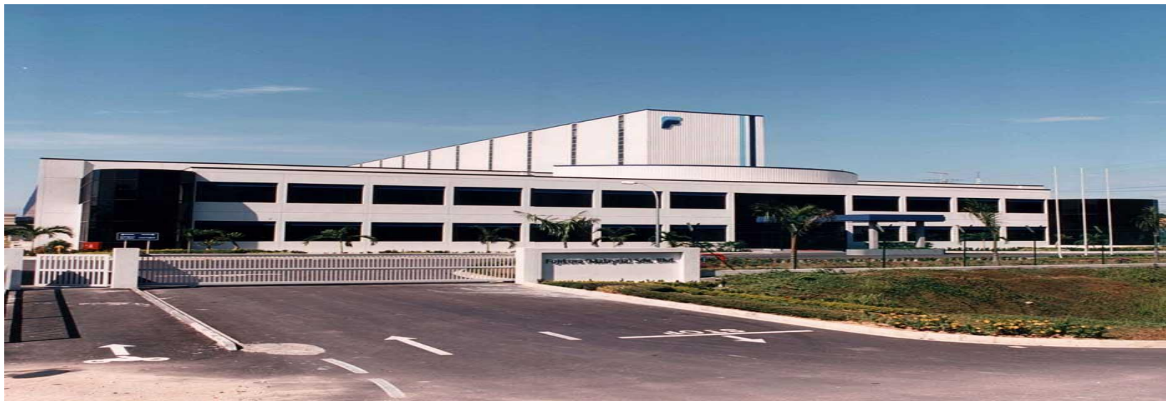
Double storey factory and administration block at Subang Hi-Tech Industrial for Fujikura (M) Sdn. Bhd.
