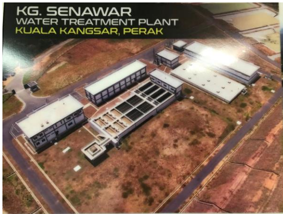
Kuala Kangsar Water Treatment Plant
