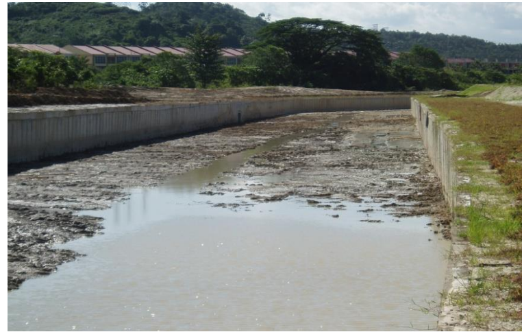
Sg. Rawang Concrete L-unit Lining in dry condition
