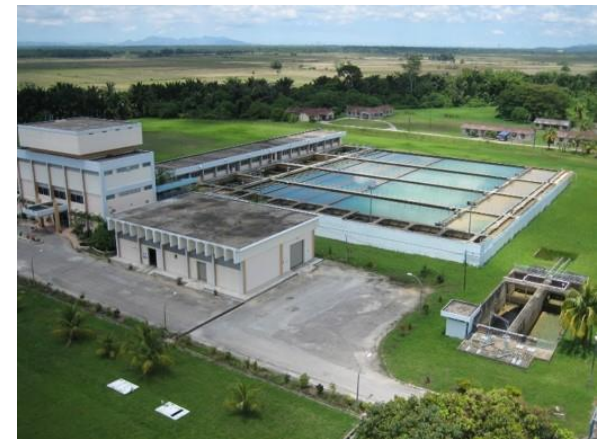
Teluk Kepayang Water Treatment Plant
